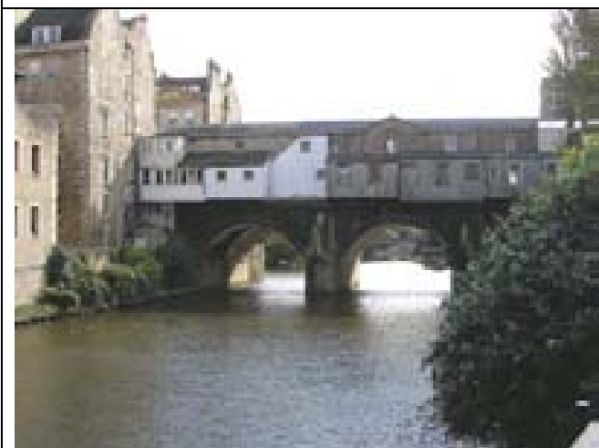
R5 Looking towards the back elevation of Pulteney Bridge.
