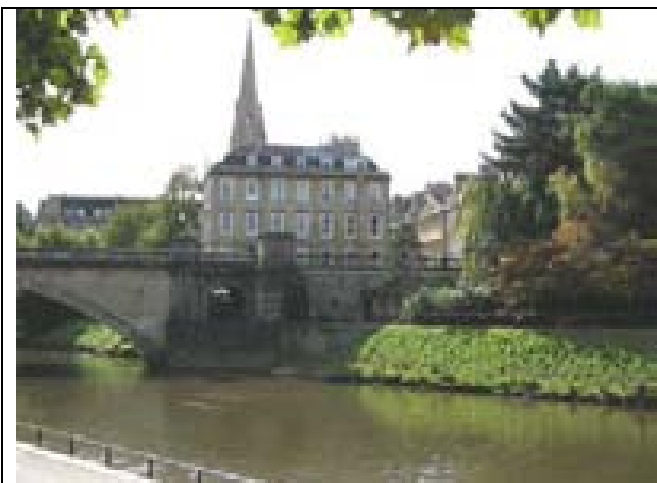
R3 North Parade Bridge looking back towards North Parade
