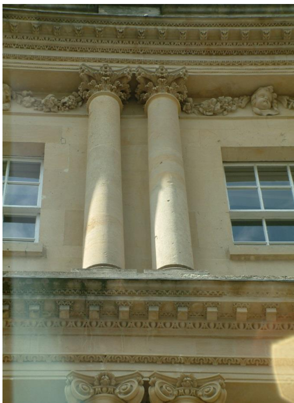
Corinthian columns, second floor level, Circus
