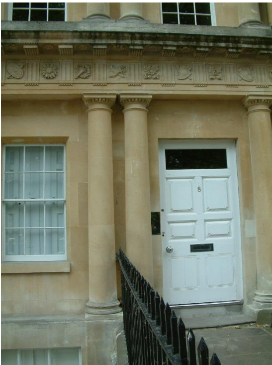
Doric columns, ground floor level, Circus
